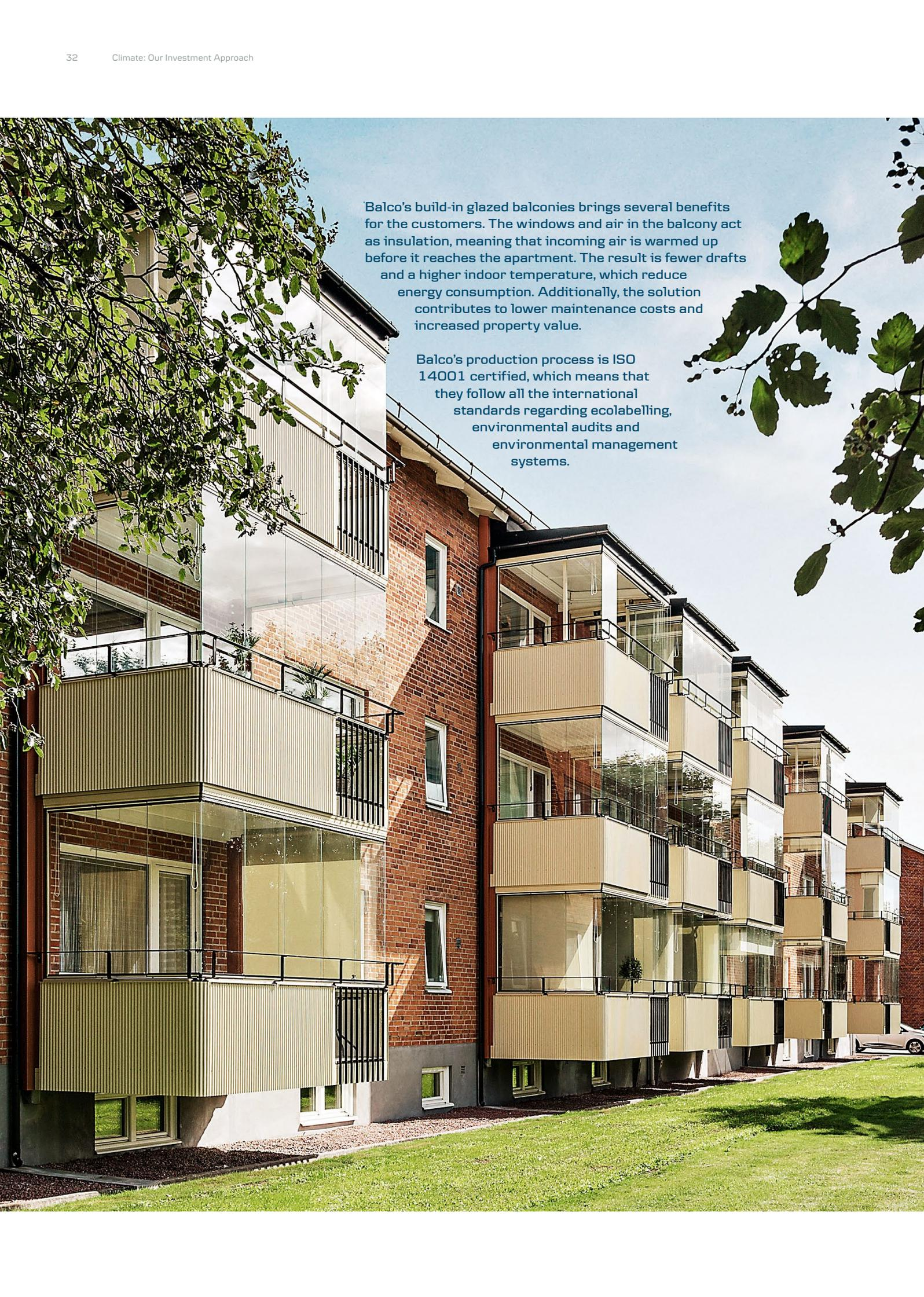
Balco's build-in glazed balconies brings several benefits for the customers. The windows and air in the balcony act as insulation, meaning that incoming air is warmed up before it reaches the apartment. The result is fewer drafts and a higher indoor temperature, which reduce energy consumption. Additionally, the solution contributes to lower maintenance costs and increased property value.
